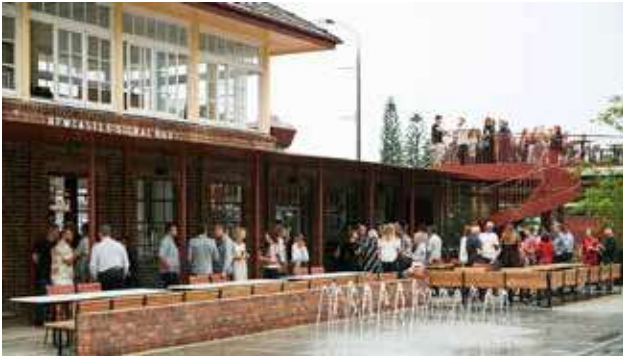
The Signal Box after 2019 after heritage restoration. (Source: Hunter and Central Coast Development Corporation)
