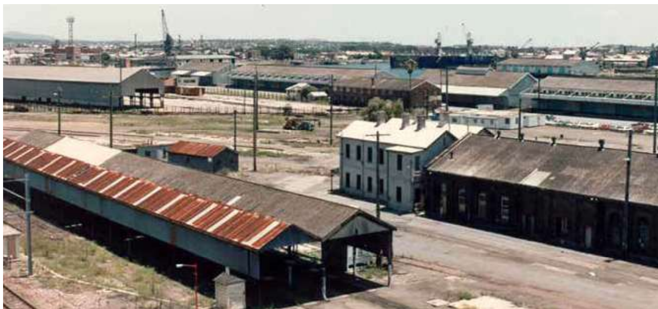
Honeysuckle before redevelopment. (Source: Hunter and Central Coast Development Corporation, Honeysuckle Celebrating 20 years )
