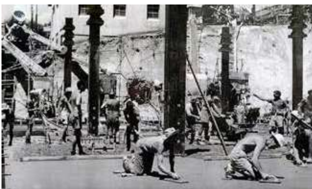
Concreters including Giusepp Suprano finish a slab at King Street car park, 1961. (Source: De Martin family)
