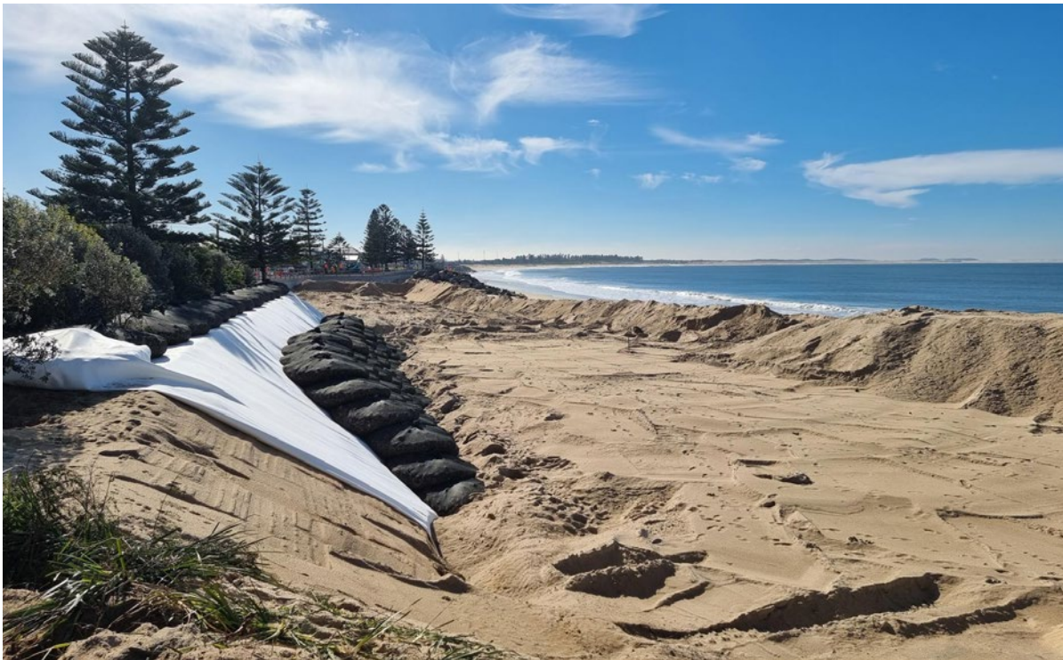
Rock bag construction. Picture supplied by Ron Boyd.
