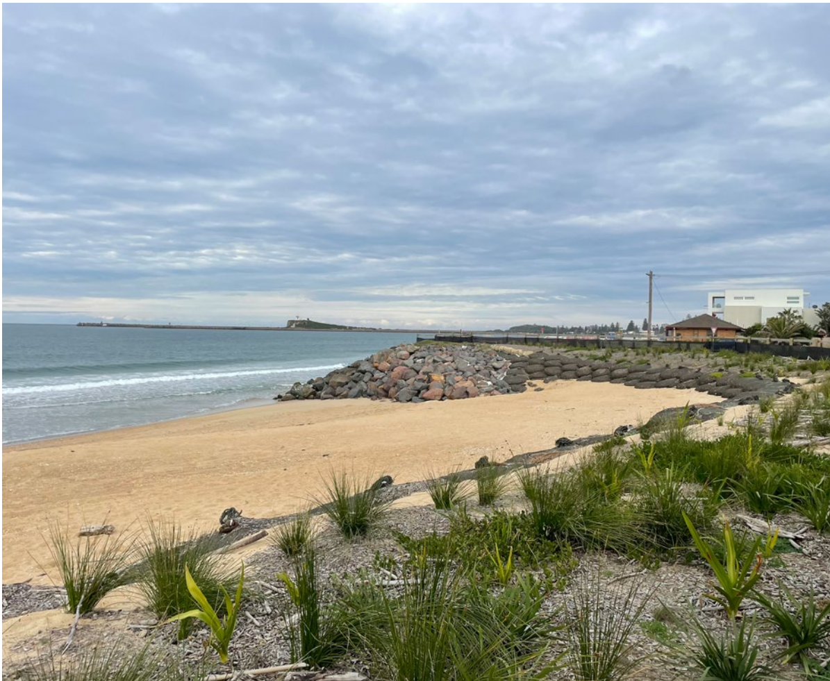
Rock bag structure at Northern end of Stockton Beach, June 2022
