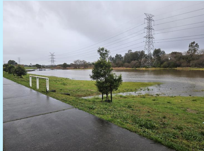
Maryland Drive during February 2025 weather event February 2025
