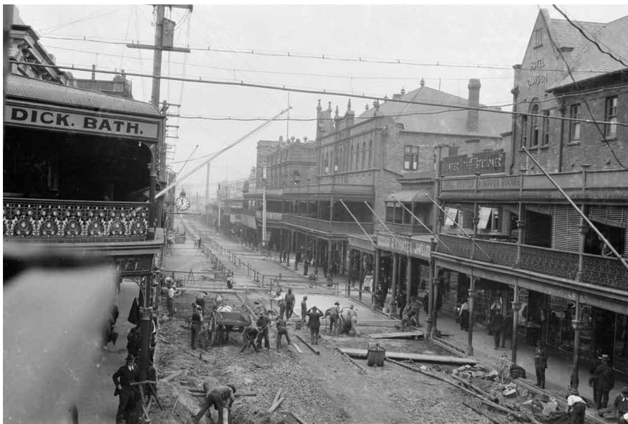
Workmen laying concrete paving, Hunter Street, Newcastle, c1921. Photographed by Sam Hood. (Source: State Library of NSW, a002809)
