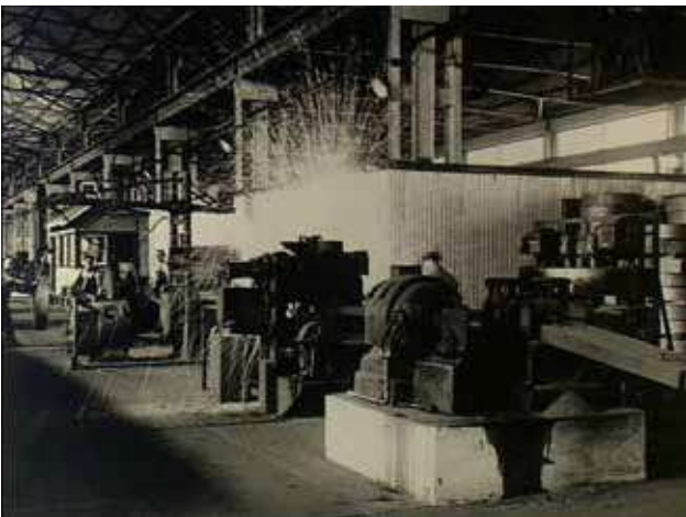
On arrival at Stewarts and Lloyds Pty Ltd tube mills from BHP Steel Works, coils of strip steel known as 'skelp' are brought to end and welded. Interior of the factory showing the operation in progress, about June 1942. (Source: Australian War Memorial, 013136)
