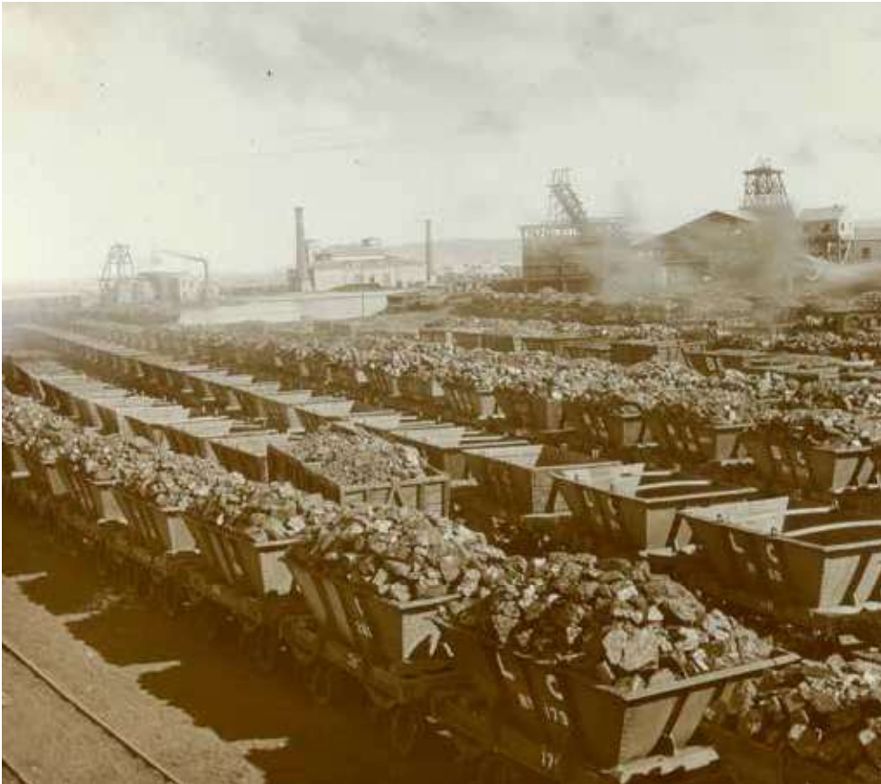
Hetton Colliery, Bullock Island, with rail trucks loaded with coal, 1875. Photograph by John Henry Harvey. (Source: State Library Victoria, http://handle.slv.vic.gov.au/10381/137239 )
